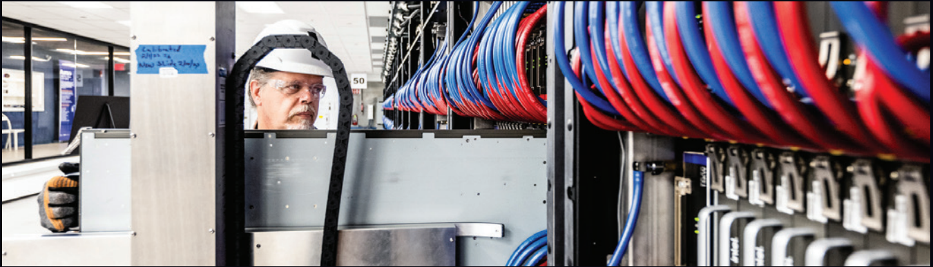
A technician uses a specialized machine to install compute blades into the Aurora system.
